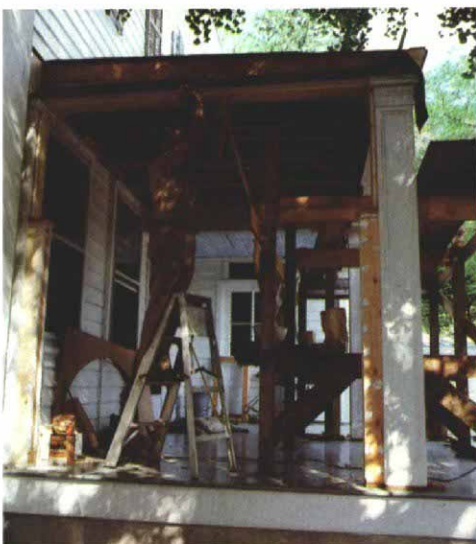
Nailing strips are fastened to the ceiling and new column sides (left) in preparation for attaching one plywood face of the entablature. Right, two identical plywood arches, fastened to nailing strips and joined with a curved soffit, complete the entablature between columns. Repeating this motif will connect the two additional columns on the finished porch, making a colonnade.
