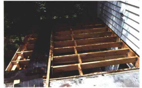
Rafters for the new roof are supported on one side by a 2x10 header bolted to the house, on the other by a girder between columns. Blocking between rafters adds rigidity.
